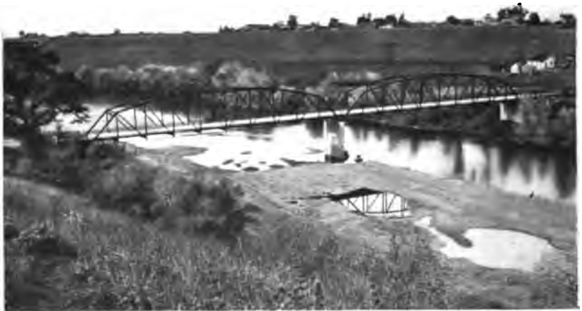
Roberts Ferry Bridge.
